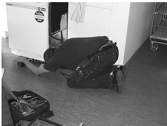
FIGURE 4.2 Installation of a dishwasher where the plumber is on his knees with one shoulder stretched forward in an extreme posture, attempting to push the machine into place. Photo: Karin Harms-Ringdahl.
