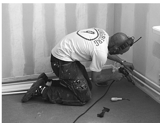
FIGURE 4.3 In carpet laying work and when welding carpet joins, the carpet fitter stands and crawls on hands and knees with his back bent and somewhat twisted and his neck slightly bent backward. Photo: Karin Harms-Ringdahl.
